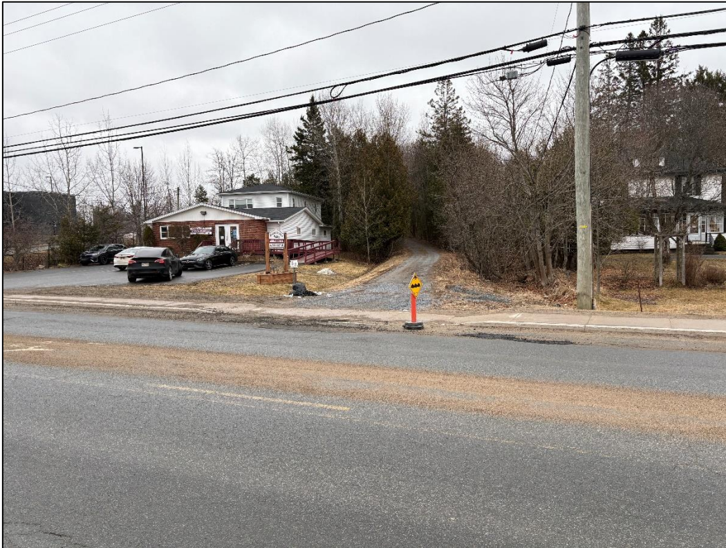
Figure 1 – View of site and adjacent veterinary clinic from Hampton Road.
