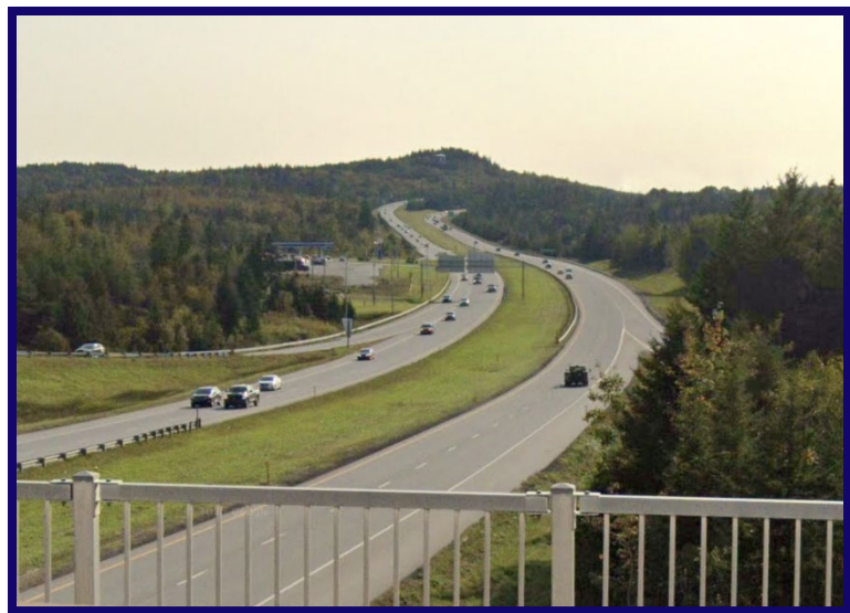
Route 1 (Mackay Highway) looking west
