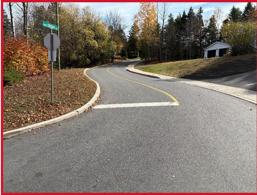
Lane Narrowing at Eriskay Drive and Iona Avenue
