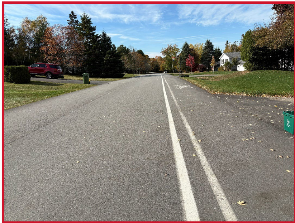
Sprucewood Avenue painted bike lane
