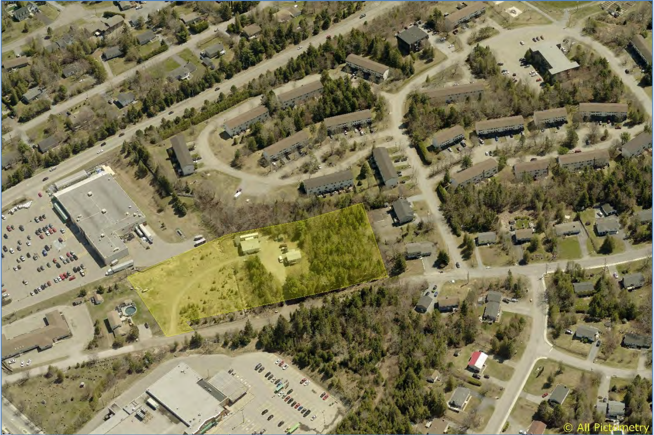
Figure 2 - Site Location off Holland Drive
