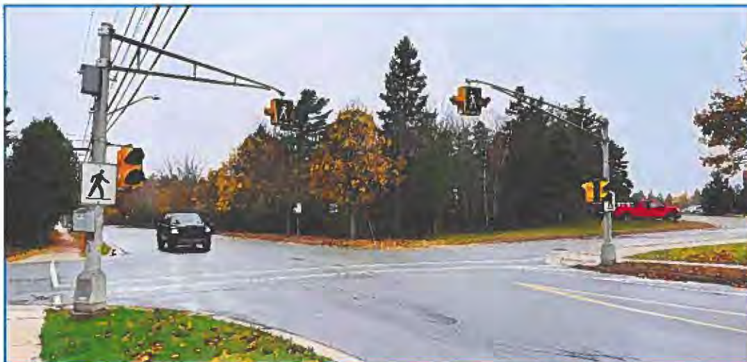
Figure 2 - Existing Overhead Crossover Signs at Hampton and Highland Avenue
