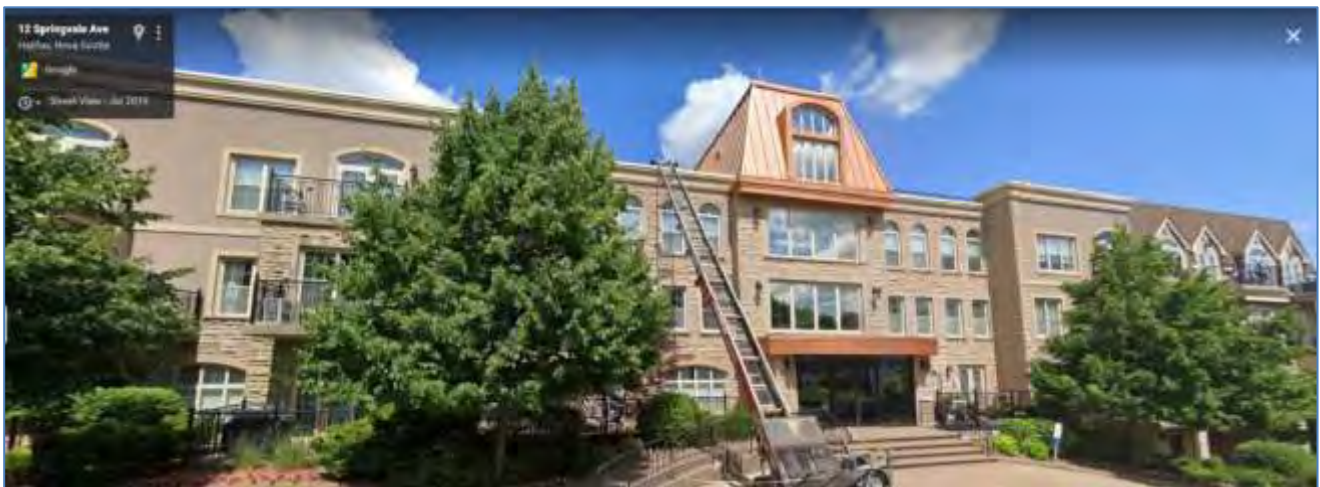
Figure 3 - Fairmont Condo Building Halifax, NS
