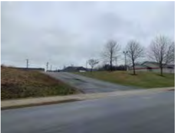
Existing Chapel Road Access
