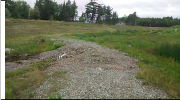
5 - At bottom of lagoon – rough areas dangerous walking
