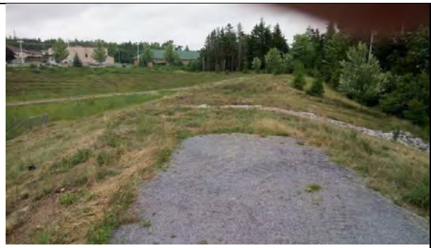
2 - Walkway ends abruptly – should be extended
