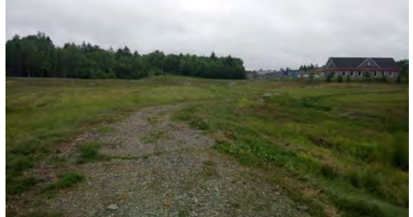
8 – Bottom walkway rough & overgrowing
