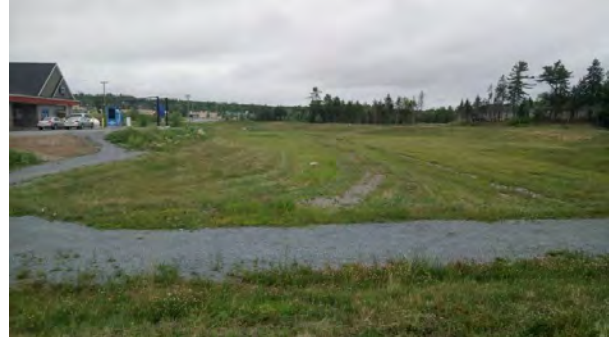
11 - North end – looking South down into lagoon – walkway overgrowing
