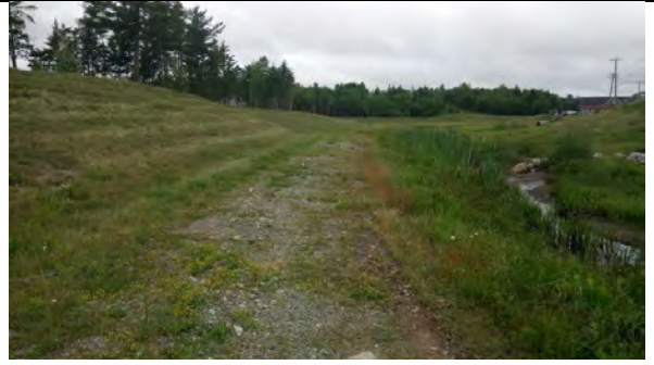
6 - Walkway over growing
