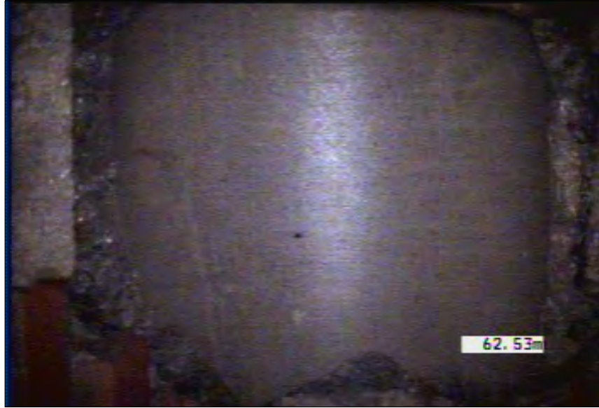
Photo: 69_69_349_A.JPG, VCR No.: 2 62.53m, Downstream Manhole, Survey Ends / CB98 Buried
