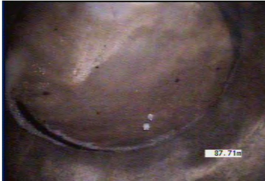
Photo: 61_61_319_A.JPG, VCR No.: 2 87.71m, Upstream Manhole, Survey Ends / Buried MH
