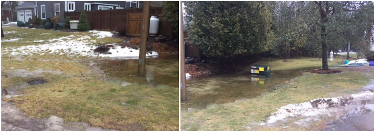
Figure 3-3: Surface Ponding Extent (right) Immediately North of 6 Brock Court and Existing Catch Basin (left)
