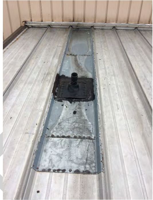
IMAGE A-015 Previous repairs to roof
