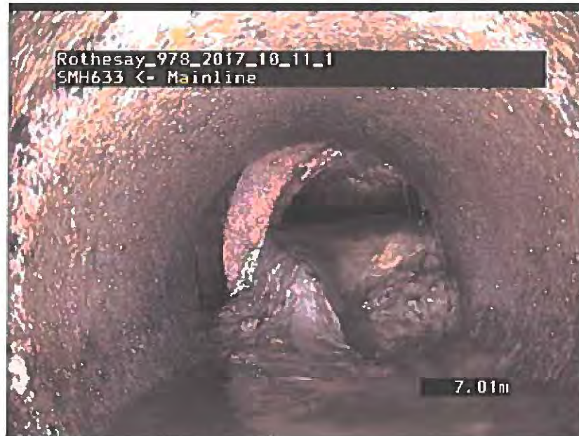
Photo: 489_489_4129_A.JPG, VCR No.: 6 7.01m, Joint Offset Large
