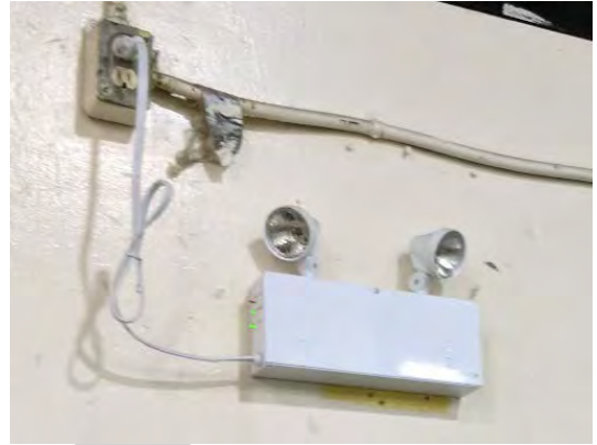
IMAGE E-026 Typical emergency lighting battery pack
