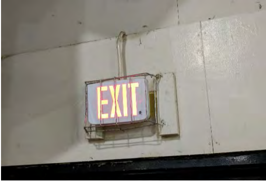
IMAGE E-025 Typical exit sign with wire guard
