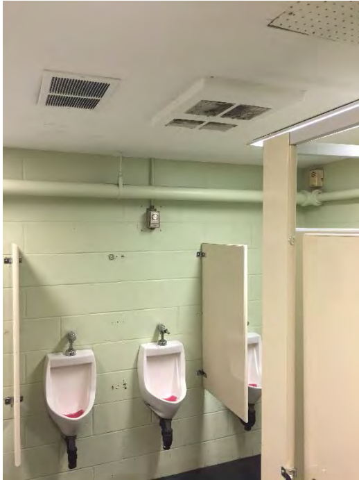
IMAGE M-021 Electric Forced Flow Heater
