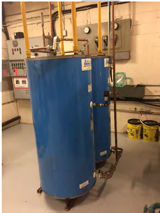
IMAGE M-015 Thermastor Tanks
