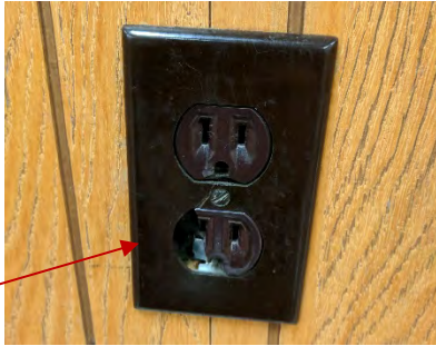
IMAGE E-015 Damaged receptacle in community room
