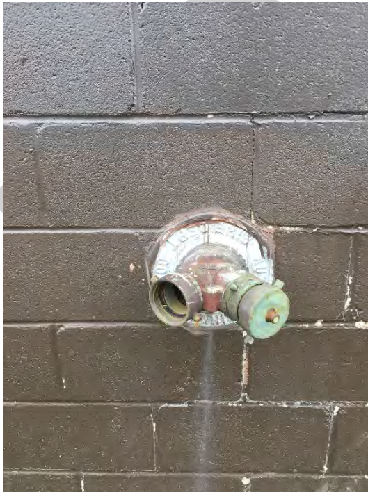
IMAGE M-011 Non-Freeze Wall Hydrant
