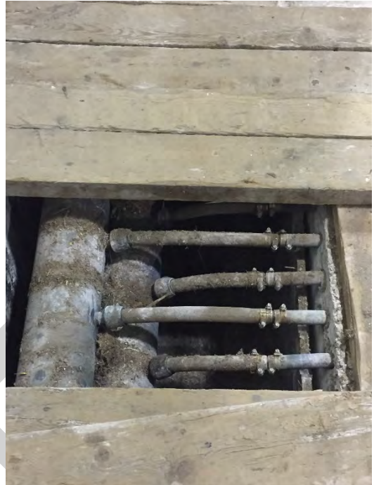
IMAGE M-034 Brine Header and Loop Branches
