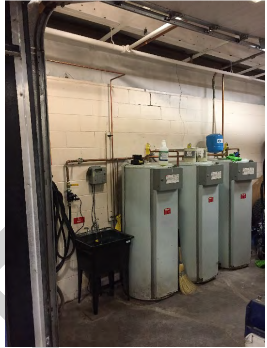
IMAGE M-014 Zamboni Hot Water Heaters
