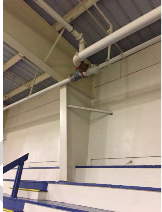
IMAGE M-018 Recently Replaced Sprinkler Pipe
