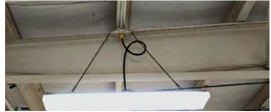
IMAGE E-016 Typical fluorescent luminaire with disconnect plug (entrance vestibule shown, others similar)
