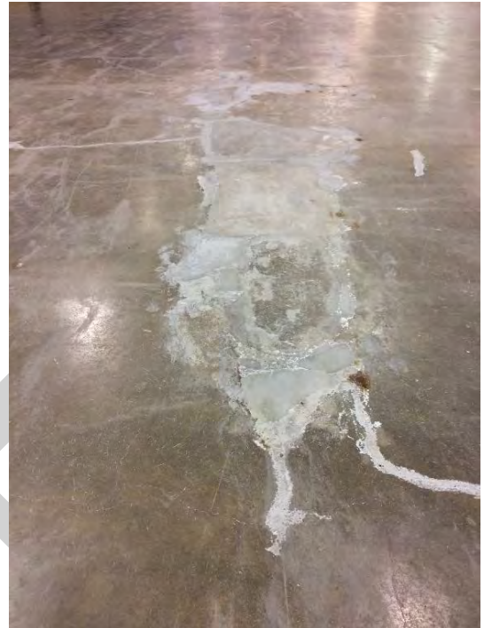
IMAGE A-002 Repair to rink slab
