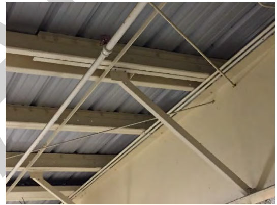
IMAGE S-008 Reinforced Roof Purlins
