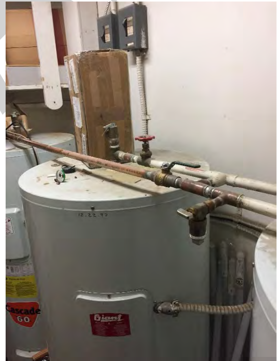
IMAGE M-012 Hot Water Heaters
