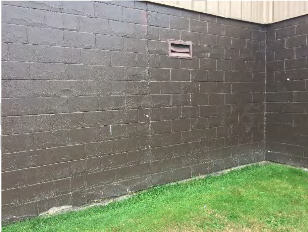
IMAGE A-009 Spalling in concrete masonry
