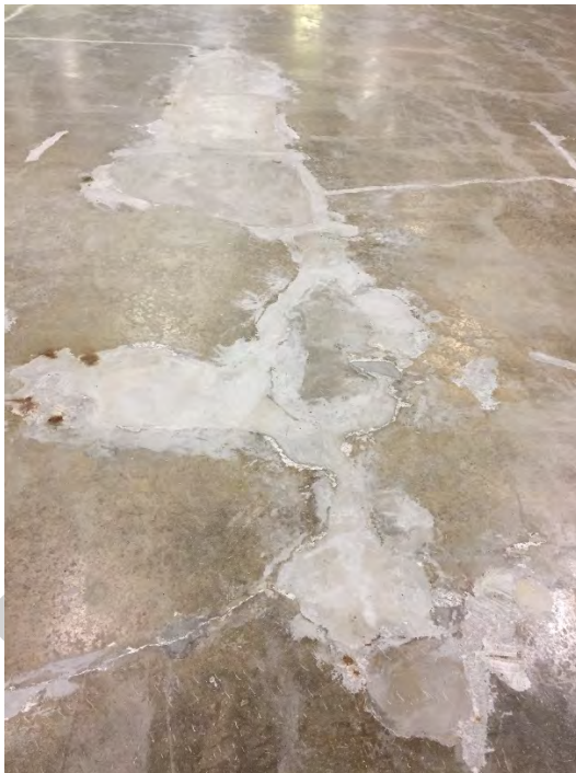
IMAGE S-007 Patched Ice Slab
