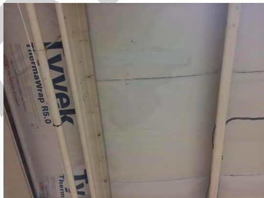
IMAGE A-037 Water infiltration above vapour barrier
