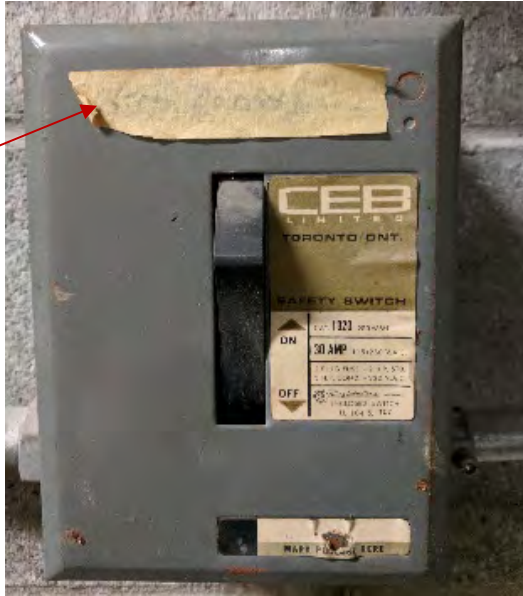
IMAGE E-005 Typical labelling with masking tape
