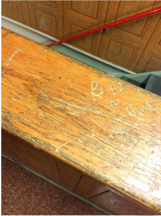
IMAGE A-005 Scratches in railing cap
