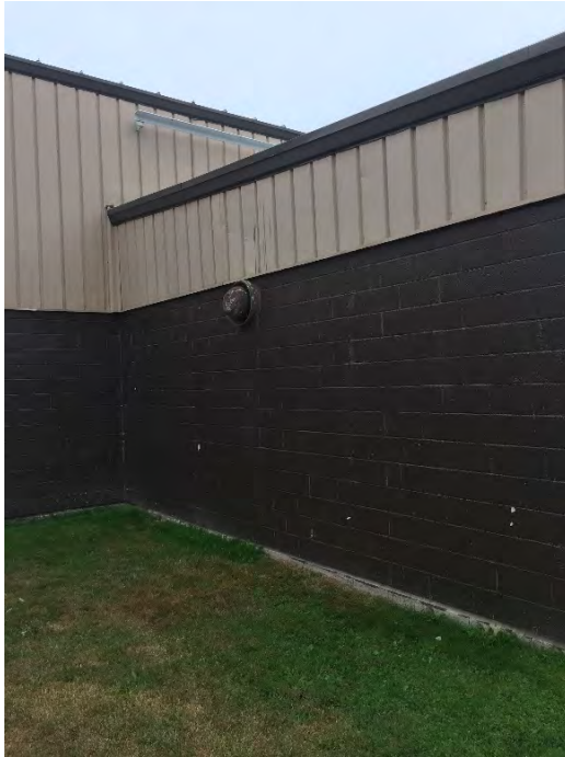
IMAGE M-025 Washroom exhaust Fan
