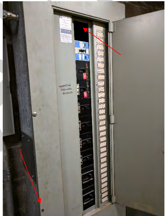
IMAGE E-004 Main 600V distribution panel with missing filler plate and fasteners
