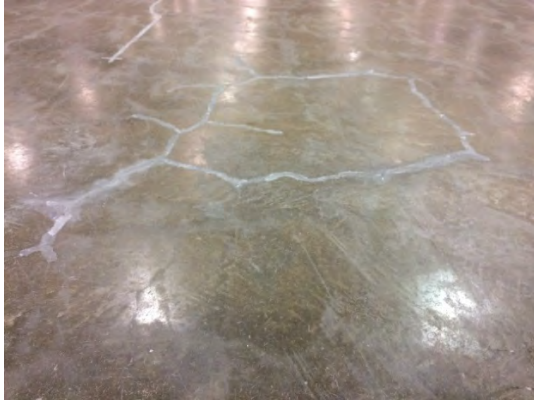
IMAGE A-001 Filled cracking in rink slab
