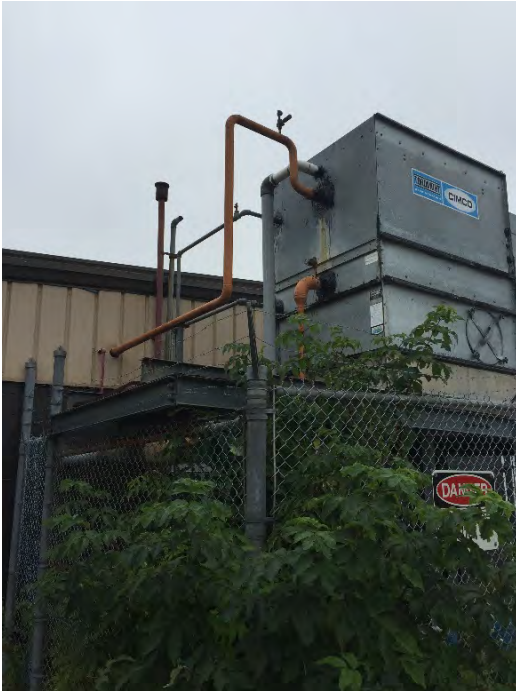
IMAGE M-033 Cooling Tower
