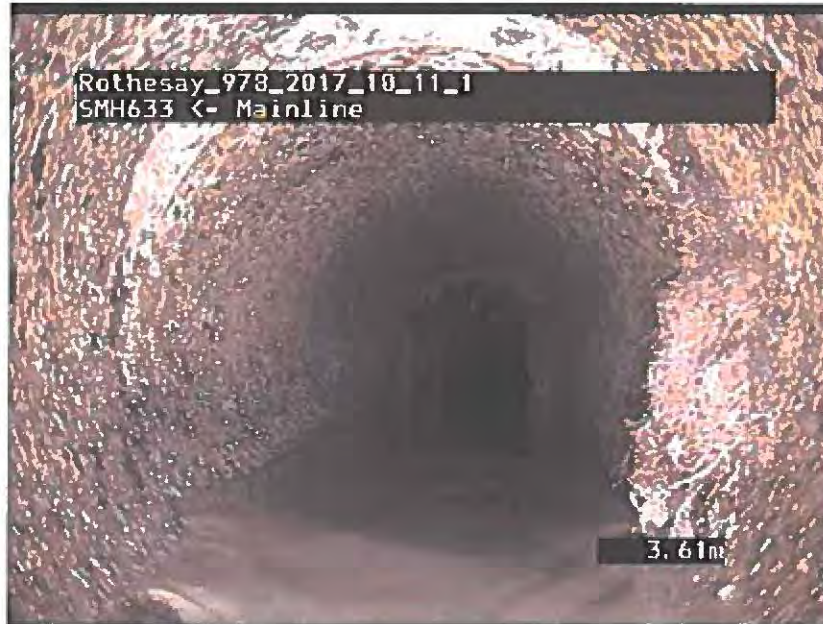
Photo: 489_489_4125_A.JPG, VCR No.: 6 3.61m, Roots Fine Joint, from 02 to 05 o'clock, within 200mm of joint: YESR
