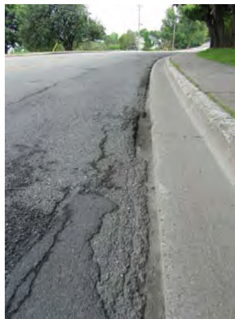
Curb and Gutter System Pavement Deterioration
