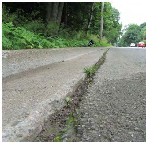
Curb and Gutter System Elevation Differential
