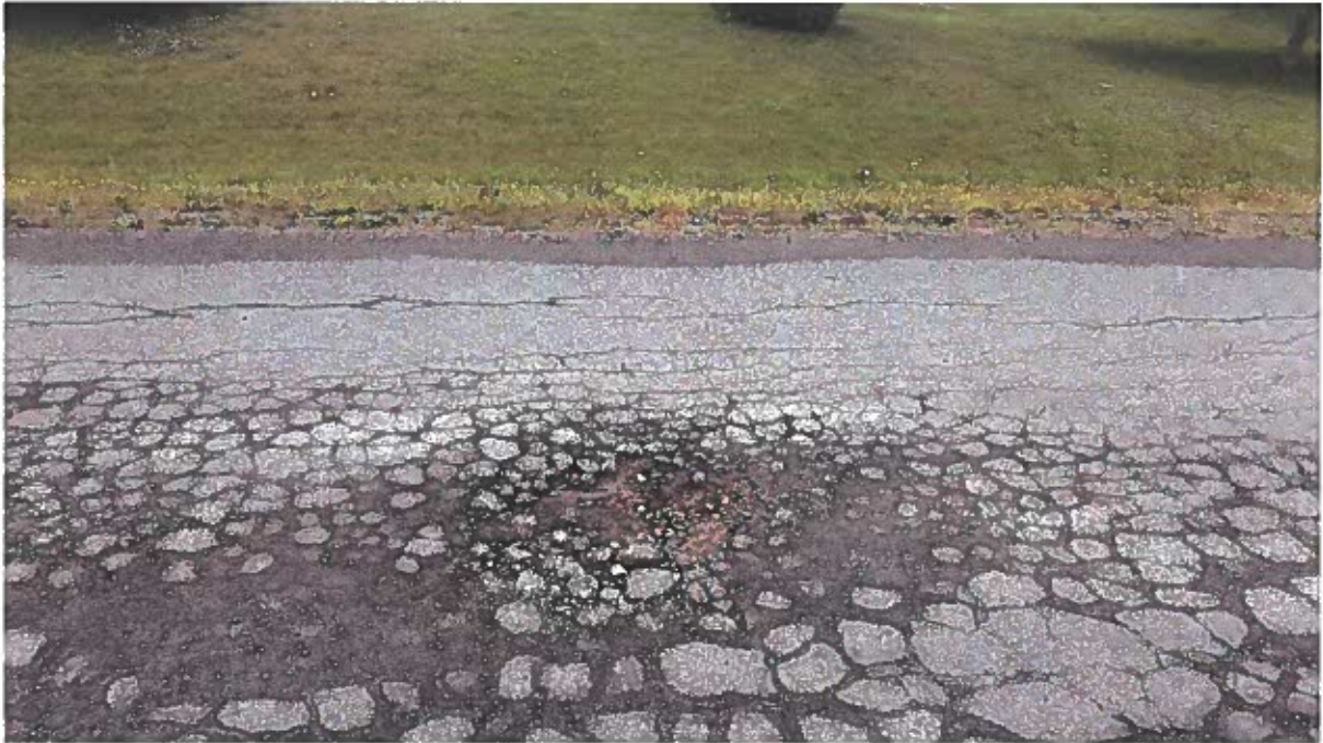
Photo 3 – South bound lane, showing map cracking and longitudinal cracking along edge
