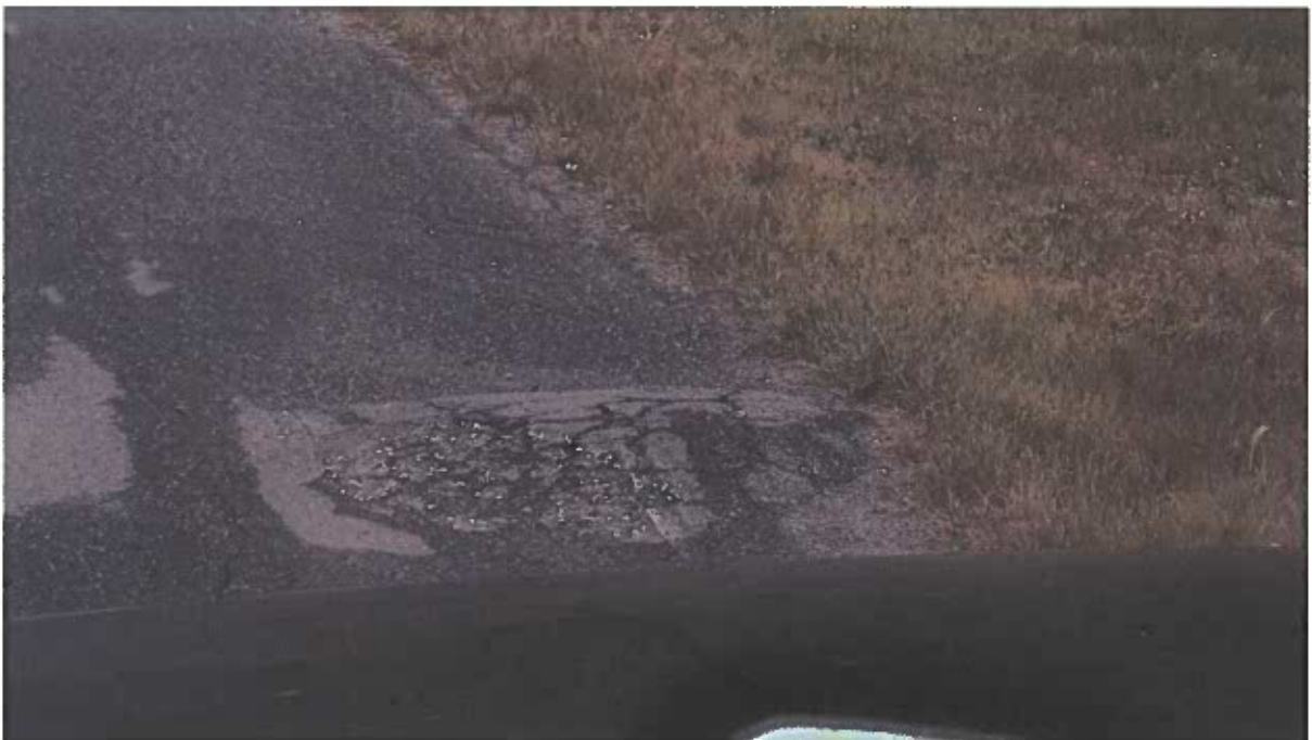
Photo 4 – Stump or boulder showing in pavement along western edge
