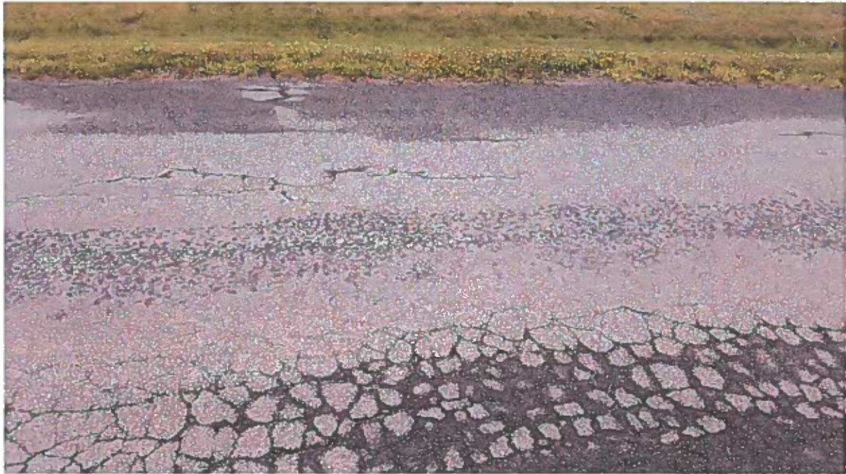
Photo 5 Severe map cracking in fore ground, bleeding in the centre and rutting associated with longitudinal in along outside of lane.
