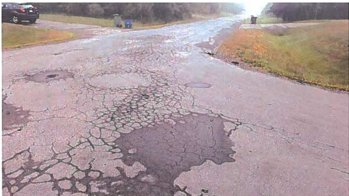
Photo 2 – looking north at intersection with Joshua Street – severe map cracking and depressions
