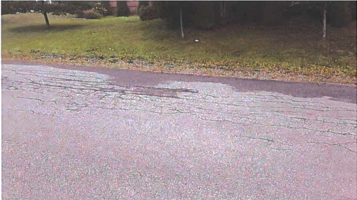
Photo 1 – Longitudinal Cracking along south bound lane, the centre of the lane is lower than the edge
