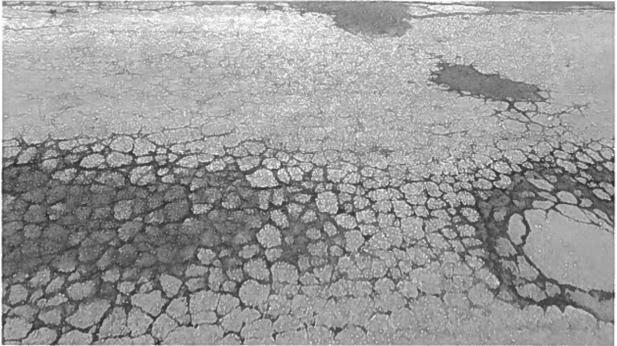
Photo 7 Severe map cracking
