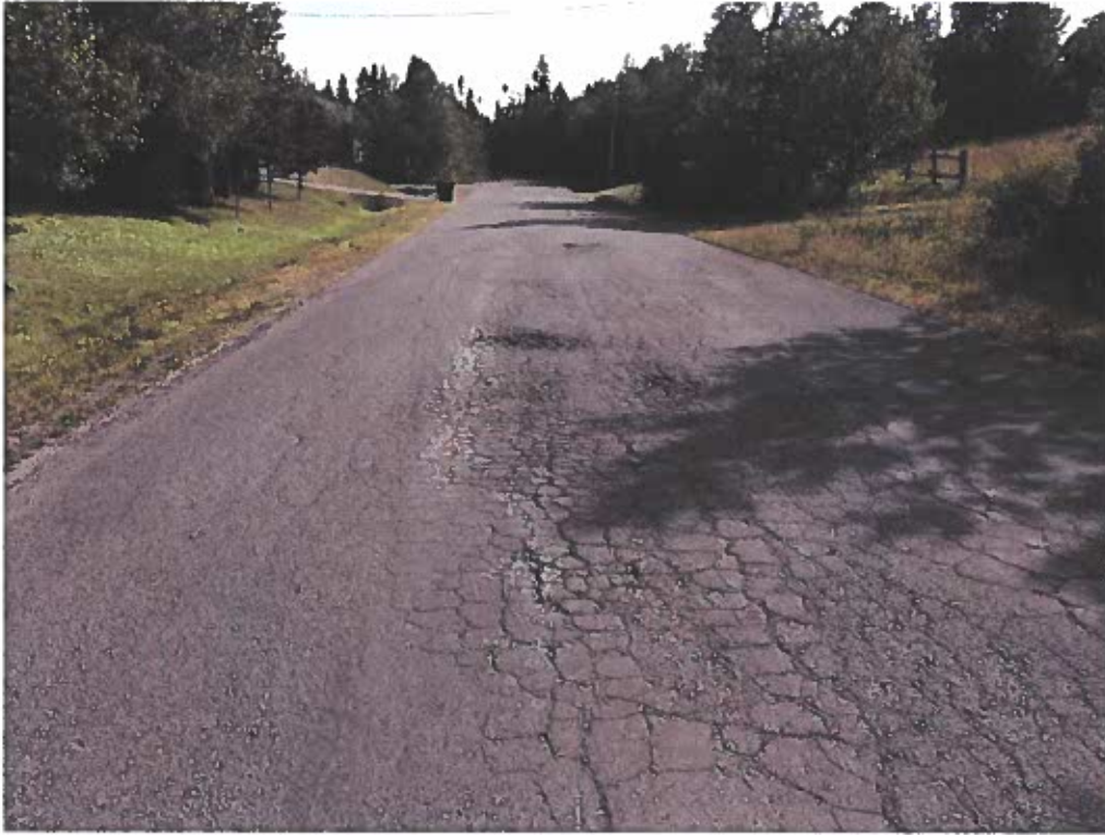
Figure 2-Observed Asphalt Cracking and Potholes on the Southern Portion of the Road. Camera Looking South.
