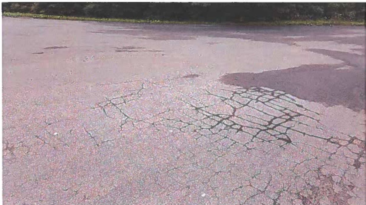
Photo 6 Northern cul-de-sac – larger sized map cracking
