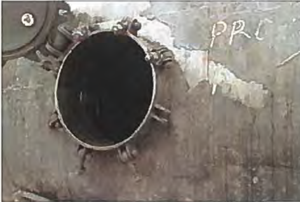
Photo 9. Missing manway tie-down
