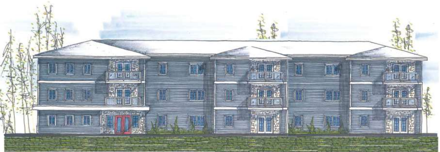
Phase 2 Rear Elevation 23 Unit Building 104 Hampton Road
